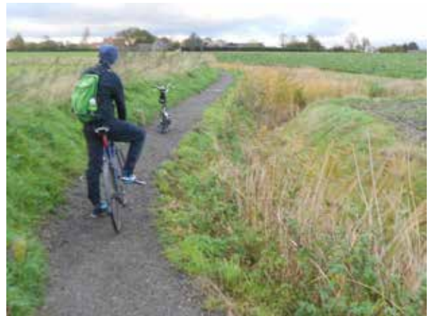
Photograph. Path pinched between stones (left) which reportedly mark property boundary, and unprotected ditch.
