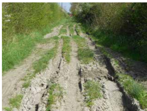
Photograph. Bridleway 12/1/2013, showing gate into Mill Drove byway, where surface becomes deeply rutted and puddled approaching Mill Road. Self-set thicket has spread from the ditches, narrowing the byway.
