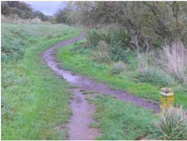
Photograph. Path leaves NCN, northward along Monk's Lode, with some space to widen and improve.
