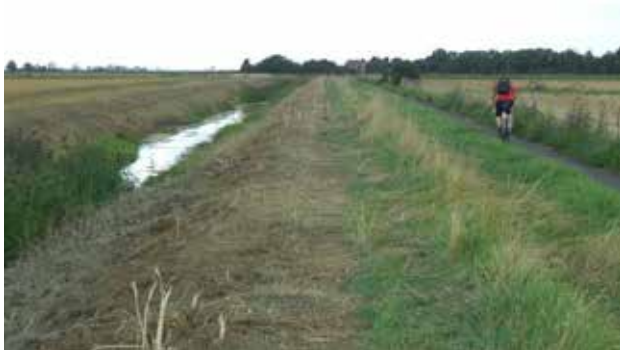
Photograph. Peterborough Green Wheel: 2 metres tarmac path behind 8 metres margin for slubbing access - work has begun. This is a good layout, but occupies a lot of land.
