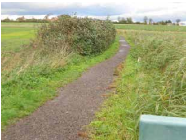
Photograph. Northward from bridge, unprotected ditch on right, seemingly space to widen path on left.
