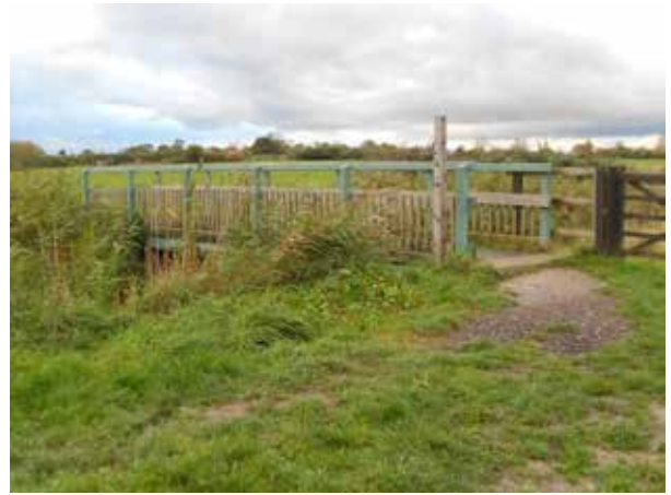
Photograph. Onwards, bridge across Monk's Lode.
