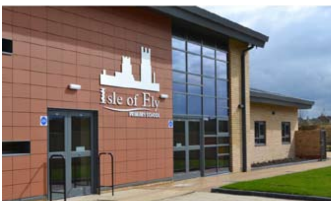
The new Isle of Ely Primary School
