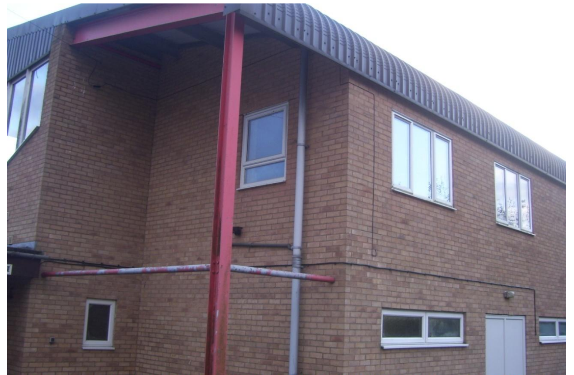
Exposed steel structure
