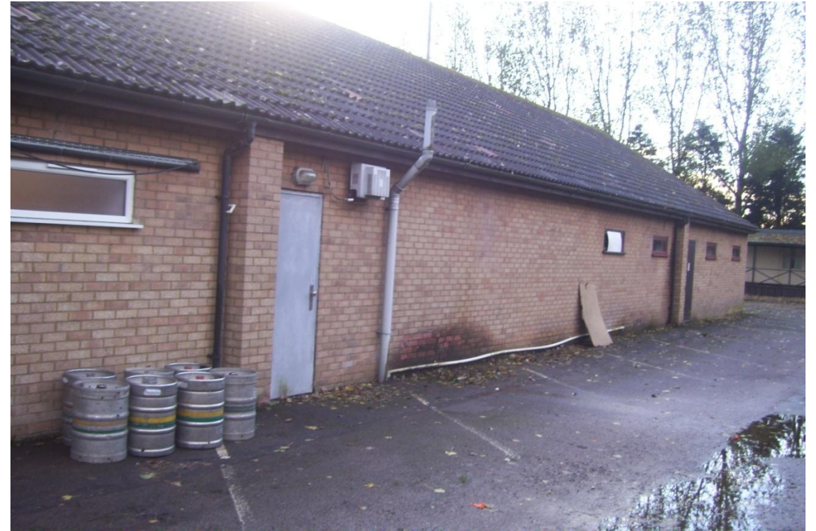
Brickwork, gutters and down pipes to the rear, note windows
