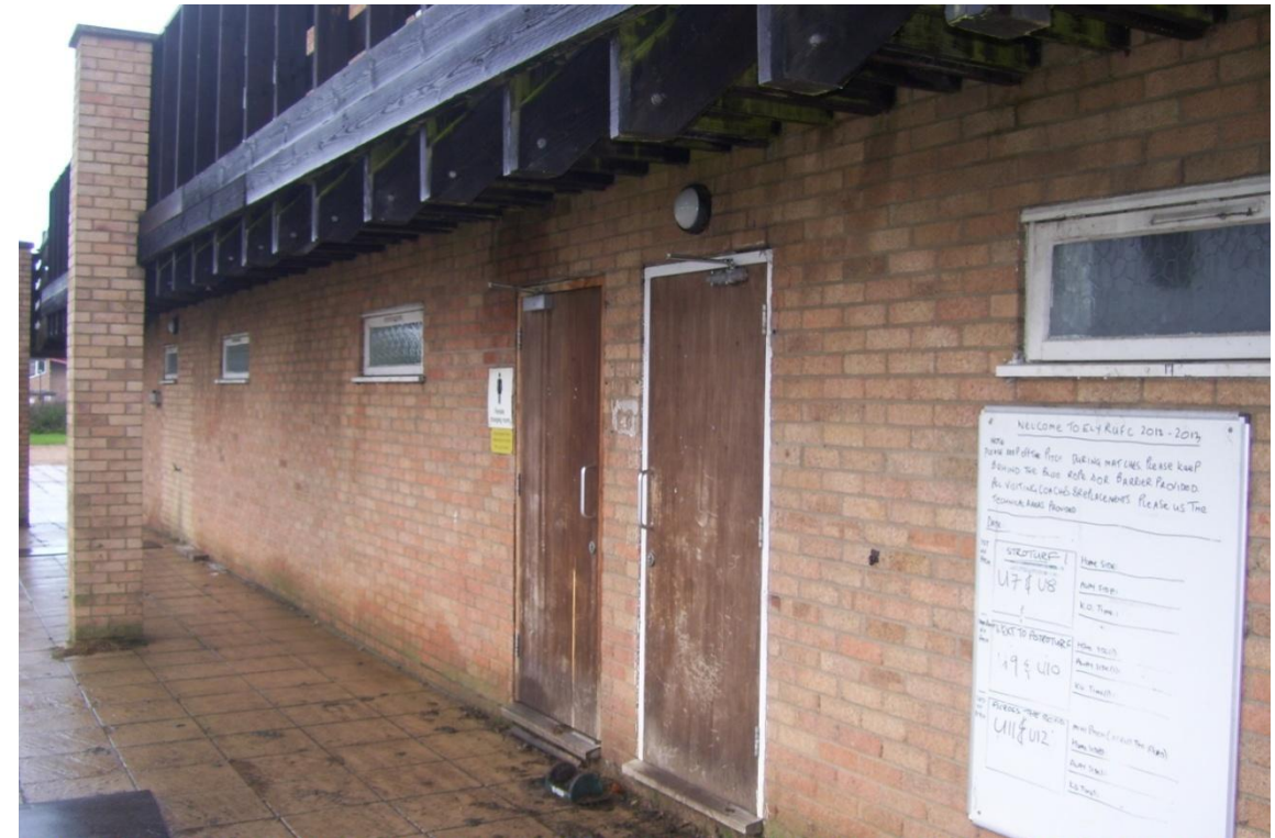
Brickwork, paving, doors & windows to EOSA club house
