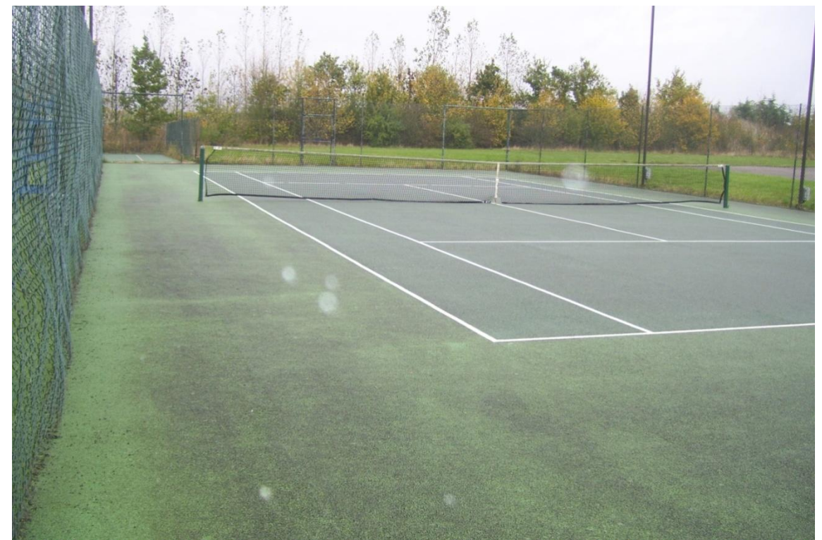
Existing Tennis Court (Worn surface)
