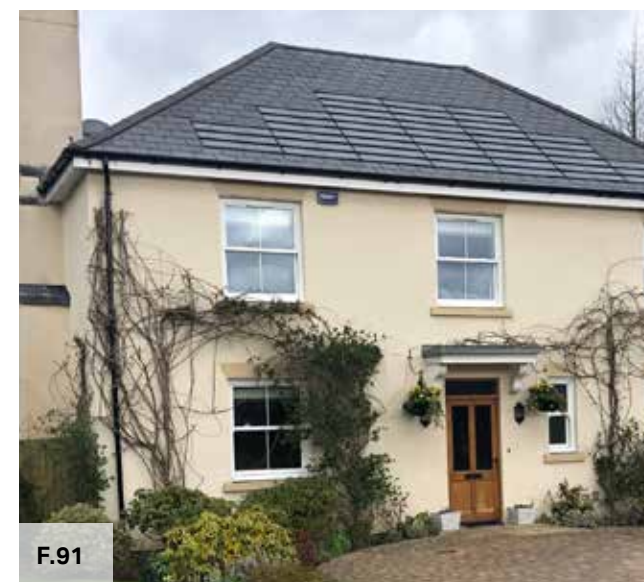
Figure 91: Use of shingle-like solar panels on a slate roof, with the design and colour of the solar panels matching those of the adjacent slate tiles.
