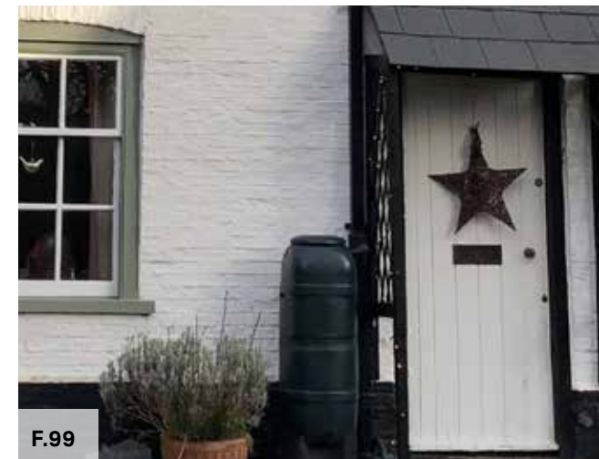
Figure 99: Examples of water butts used for rainwater harvesting in Cambridgeshire
