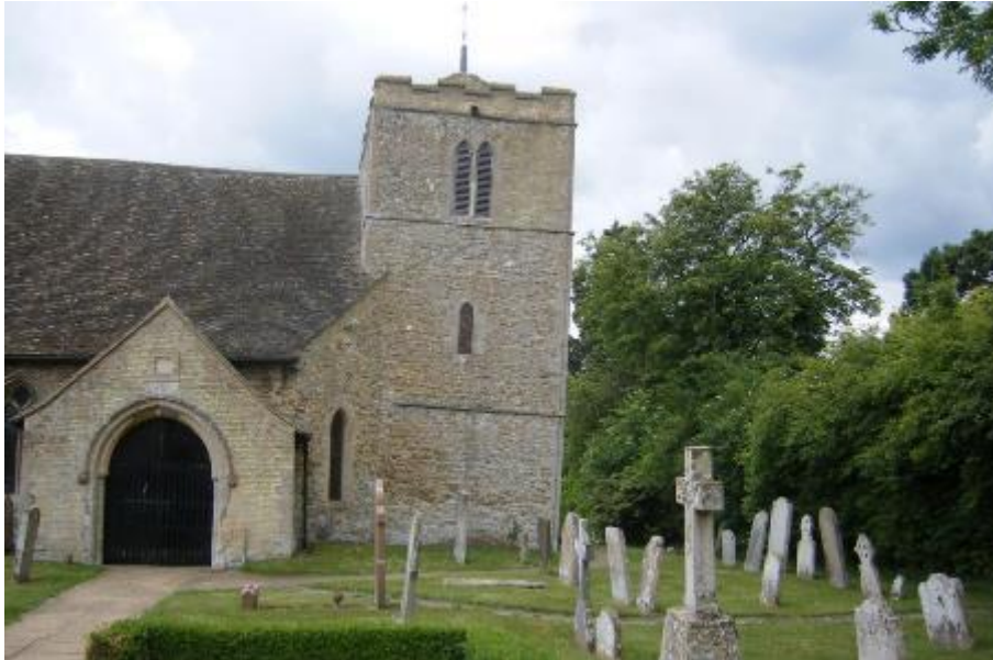
© East Cambridgeshire District Council
