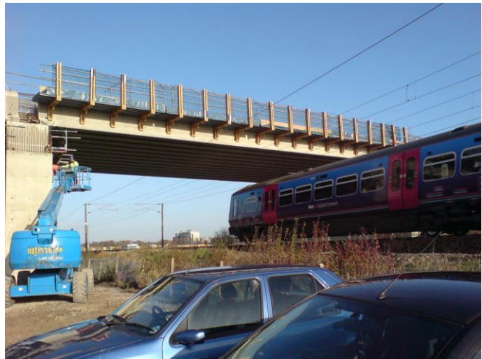
Construction of Busway bridge over railway at Addenbrooke's
