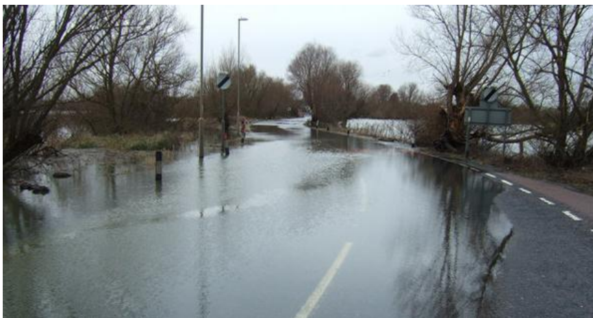
Flooding on the A1123 at Earith
