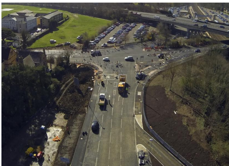
The junction of Brampton Road with Huntingdon Station access and the new Huntingdon West of Town Centre Link Road (Edison Bell Way), which is opening up land for development.
