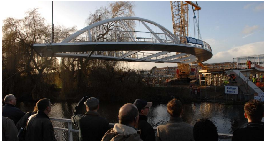
The Riverside Bridge in Cambridge, which was part funded by development
