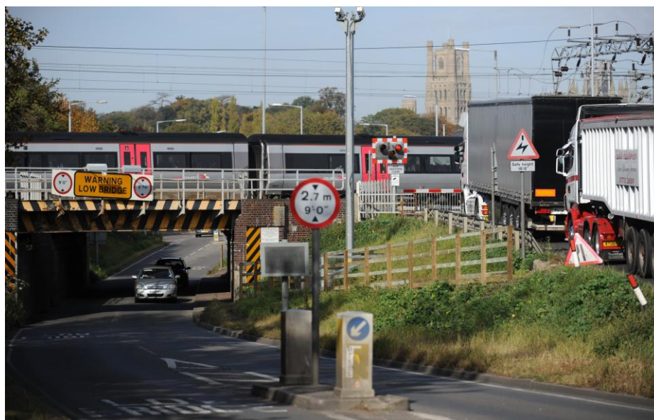
The low bridge and level crossing on the A142 to the north of Ely Station.
