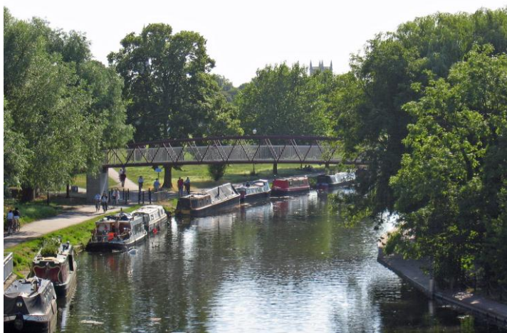
The Cutter Ferry pedestrian / cycle bridge in Cambridge
