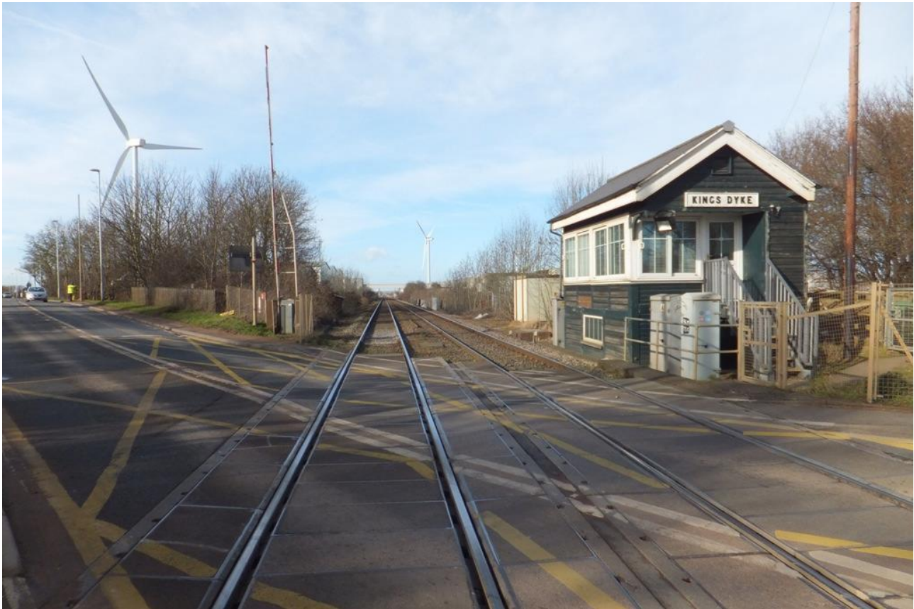
The Kings Dyke level crossing
