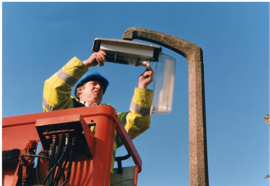
Street light maintenance
