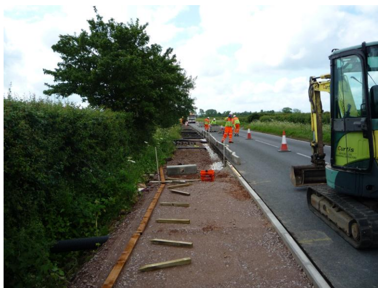
Construction of the Swavesey to Buckingway Business Park cycle route
