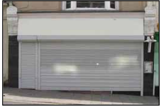
Roller shutters creating a dead frontage with no visual transparency into shop
