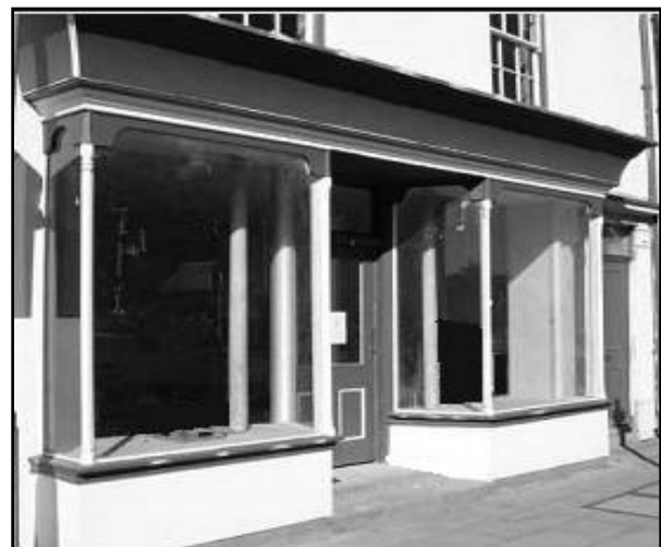
Well designed entrance way:
