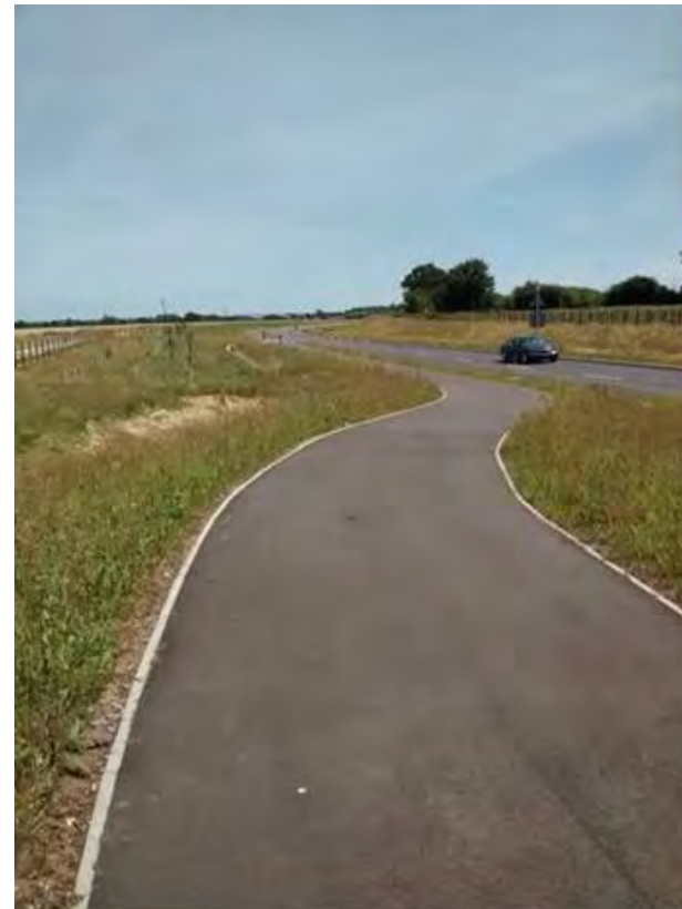
Figure 3.5 Smooth, tarmac surface, accessible for all non-motorised users
