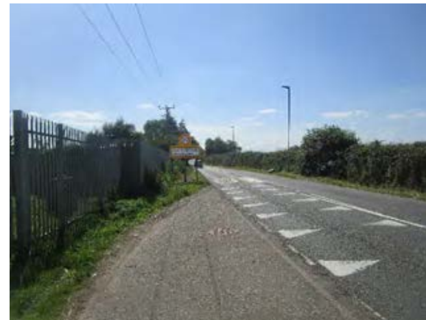
Figure 7E 6.1 A new safe crossing is needed in this area (view towards A1123).
