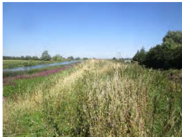
Figure 7D 5.1 View of the bank top from near the A1123 looking north-east.
