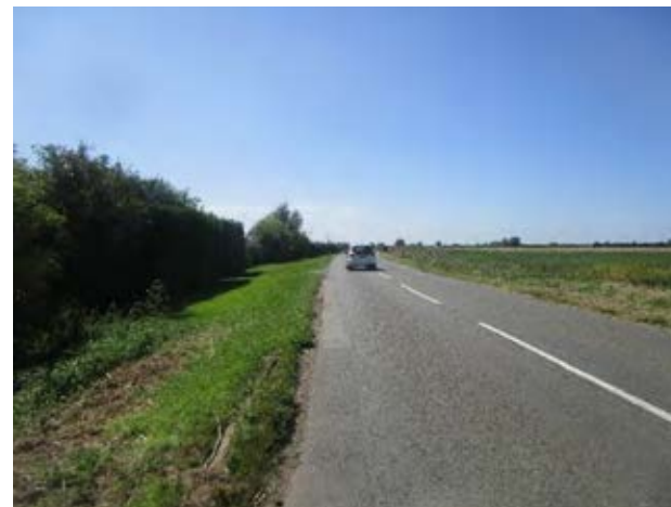
Figure 7E 9.11 View along B1381 towards Earith A new path would need to be in the verge to the left set back as far as possible.
