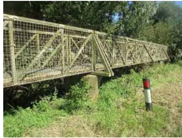
Figure 7A.16.3 View of structure in dry conditions.
