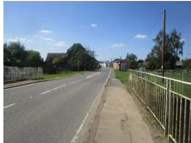
Figure 7D 3.1 View towards Earith of the bridge and footway. There is little scope for reallocating road space.
