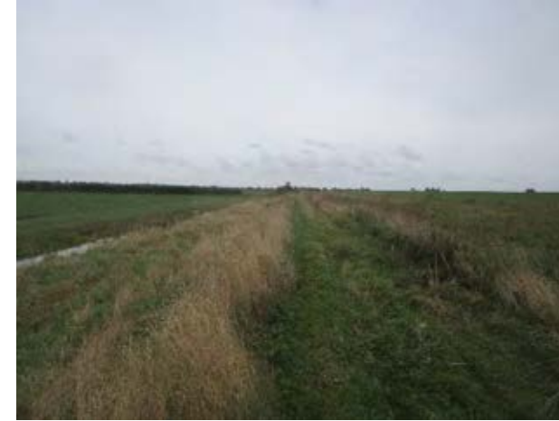
Figure 7A.7.5 View along flood bank towards Sutton with flooded field to right and watercourse to left showing potential route on field to left.
