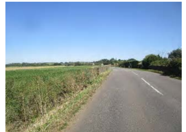
Figure 7E 7.3 View along B1381 towards Earith. A new path would need to be in field to the left for this option.
