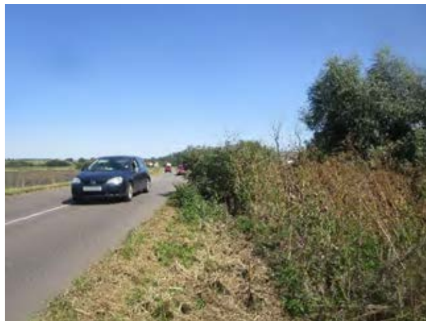
Figure 7E 8.1 View along B1381 towards Sutton A new bridge would need to be to the right of the road and the existing road
