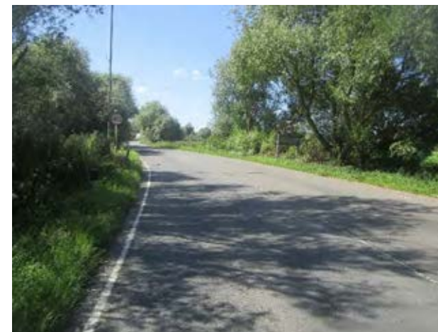
Figure 7D 4.1 View of the A1123 looking towards Earith. A causeway would have to be in fields to the right.
