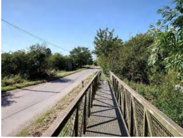
Figure 7A.16.5. The bridge/ causeway connects to higher ground at each end.
