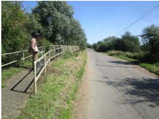
Figure 7A.16.6. The bridge/ causeway connects to higher ground at each end.
