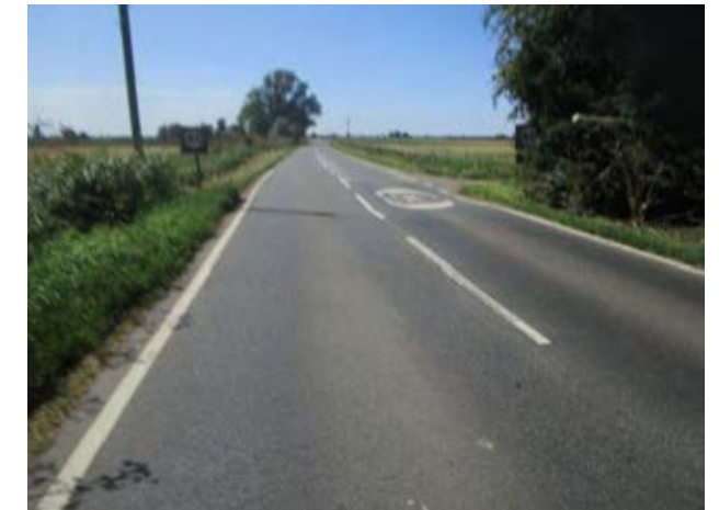
Figure 7D 8.1 A gateway feature and safe crossing is needed in this area on the edge of Sutton. The view is towards Earith and for this option a new path would need to be on field edges on the right beyond the trees.
