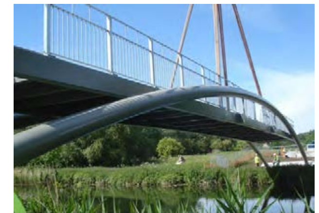
Figure 7D 4.1 View of the Willow Bridge crossing the River Great Ouse at St Neots. For a route following the A1123 there are two major rivers to cross.
