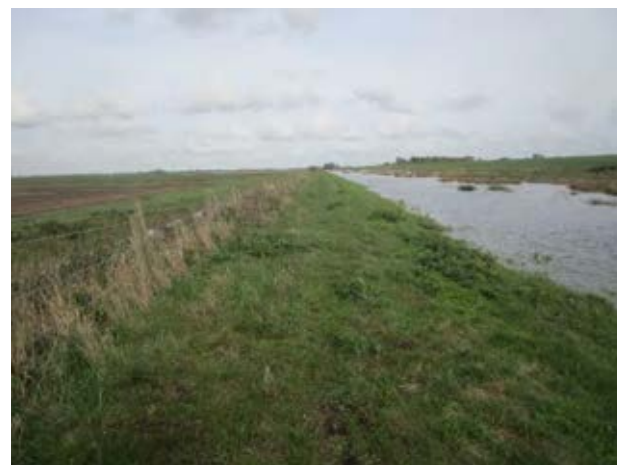
Figure 7A.7.3 View along flood bank towards Sutton with flooded field to right and watercourse to left showing potential route on field to left.
