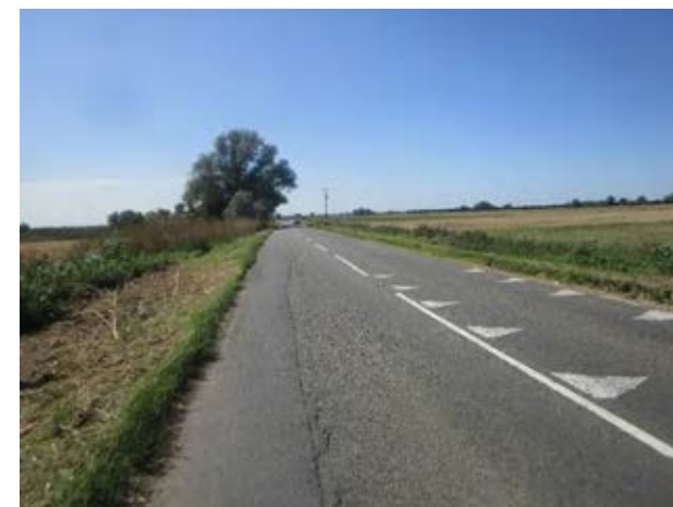
Figure 7D 7.2 View along B1381 towards Earith. For this option a new path would need to be in field edges to the right and would have to finish near this area.
