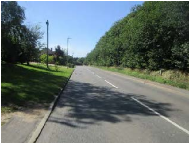
Figure 7D 9.1 View of The America towards Earith. The removal of centre lines and new cycle lanes is one option to consider, but traffic speeds are a concern.
