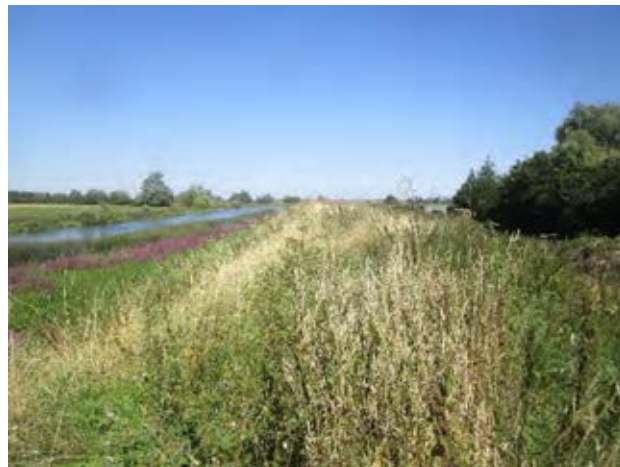
Figure 7E 5.1 A new path would need to ramp down from this position towards the trees on the right.
