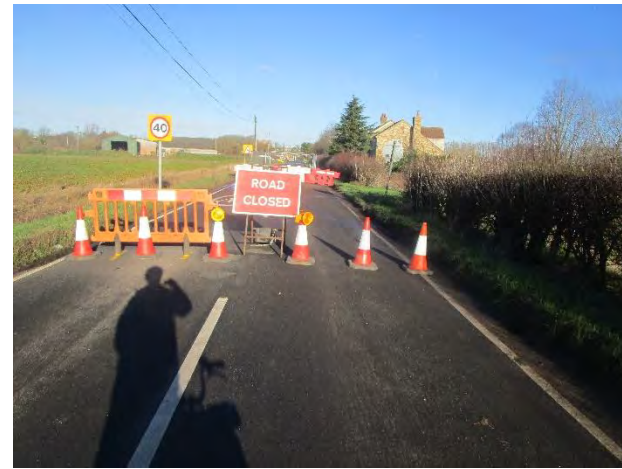
Figure 5.2.2– Twenty Pence Road closure, near Wilburton
