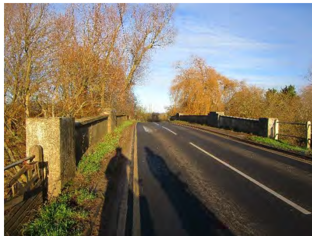
Figure 5.2.1 – Twenty Pence Road bridge
