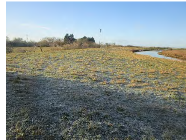
Figure 7C9.4 River Great Ouse flood bank view towards Cottenham Lode from Twenty Pence Road. A path here looks achievable, subject to consent.
