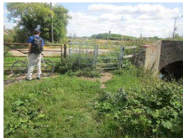
Figure 7C6.5 The route meets Lockspit Hall Drove with a kissing gate that needs replacing with a cattle grid and gate or similar.
