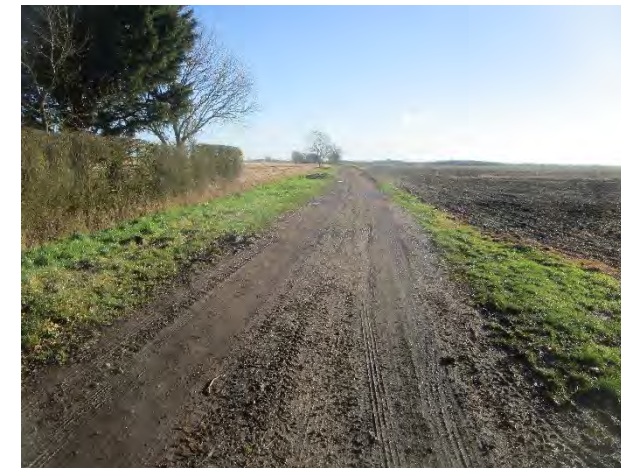
Figure 7C15.1 Cut Bank in one of the better parts.
