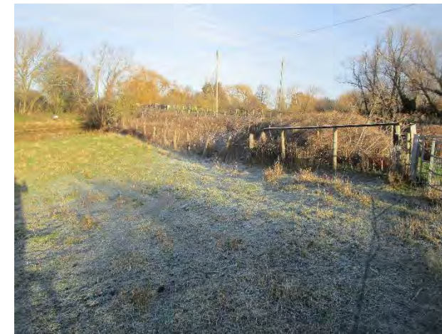
Figure 7C9.5 River Great Ouse flood bank view towards Twenty Pence Road. Improved access is needed here.
