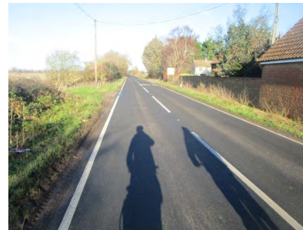
Figure 7C11.2 Twenty Pence Road north of the river bridge with properties to the right, making path construction on the right challenging.
