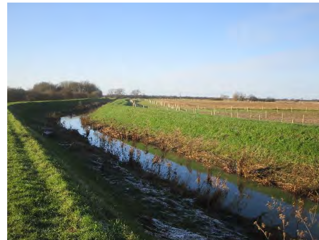
Figure 7C8.4 View across Cottenham Lode towards Cottenham. A field path near the opposite bank would be needed for this option.
