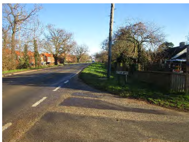
Figure 7C16.1 Millfield Lane/ A1123 junction.
