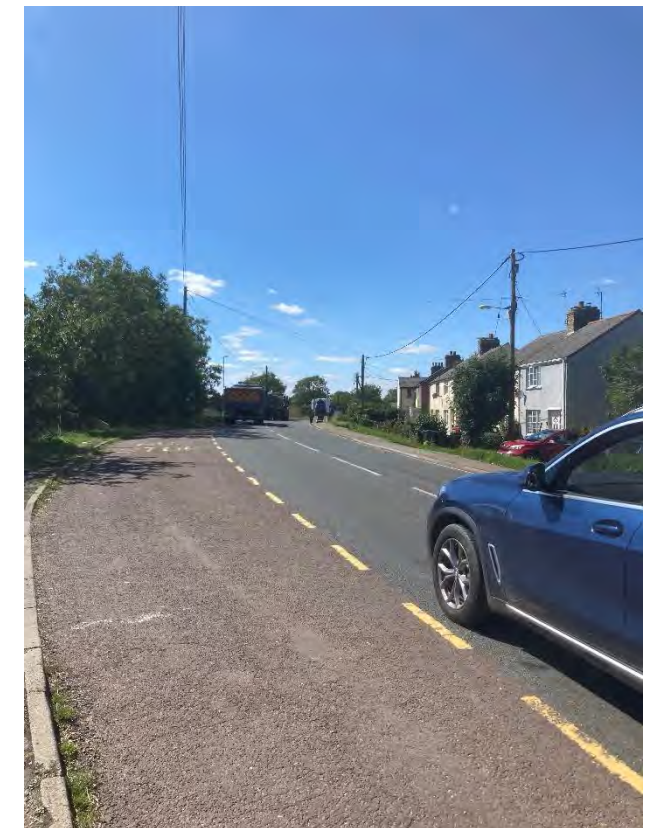
Figure 5.2.6 – A1123 slightly west of Wilburton centre
